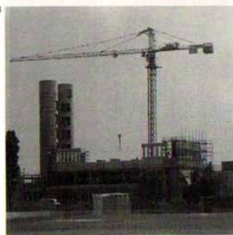
Its concrete, class Rck 350 kg/cm<sup>2</sup>, was additized with a superfluidizer and with an expansive agent to counteract thermal shrinkage and a part of the hydraulic shrinkage.
